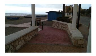
All entrances to the plots are accessible by means of a level or very gently sloping ramp with tactile paving.
